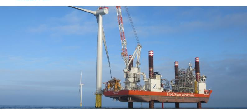
Fred. Olsen Windcarrier joined the Galloper installation project midway in 2017 to support timely completion for client Siemens Gamesa Renewable Energy (SGRE). The scope of work included delivering a fully mobilised vessel, with marine crew for transport and installation.
